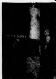
Shrinking a Liner with Dry Ice, at -110^{\circ} F., before Sliding into the Cylinder, Some of which work at Pressures of 22,500 lb. per Sq. In.
